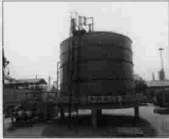
Low Rate Bio Filter (LRBF)
