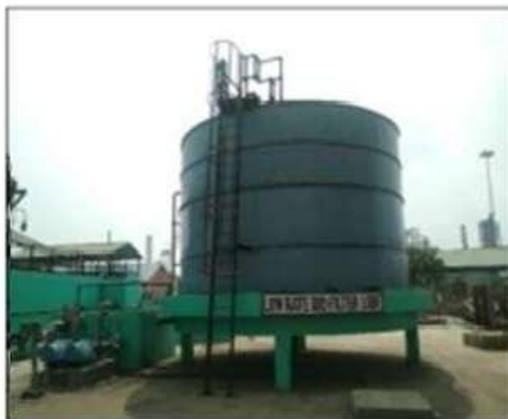
Low Rate Bio Filter (LRBF)
