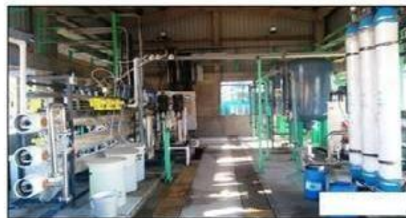
Figure 6: Photograph of Existing RO plant
