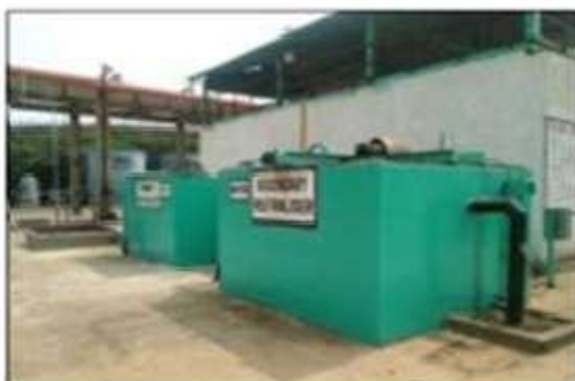
Primary & Secondary Neutraliser
